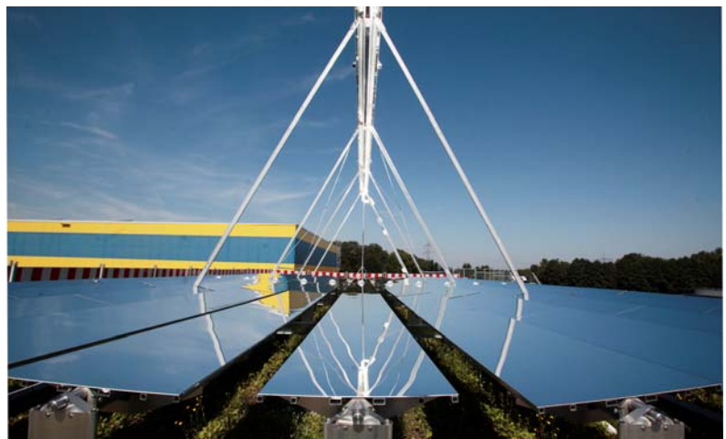
Solar thermal pilot plant in Umkirch near Freiburg, Germany. In the research project "AgroKühl", solar thermal energy is utilized to power cold rooms for food and medicines. ©Kramer GmbH
